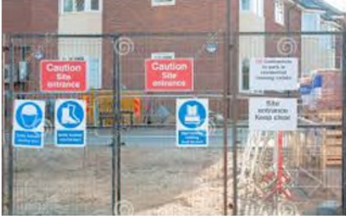
Example of signage at entrance to site
